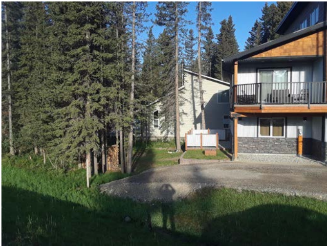
Dwelling and adjacent landowner
