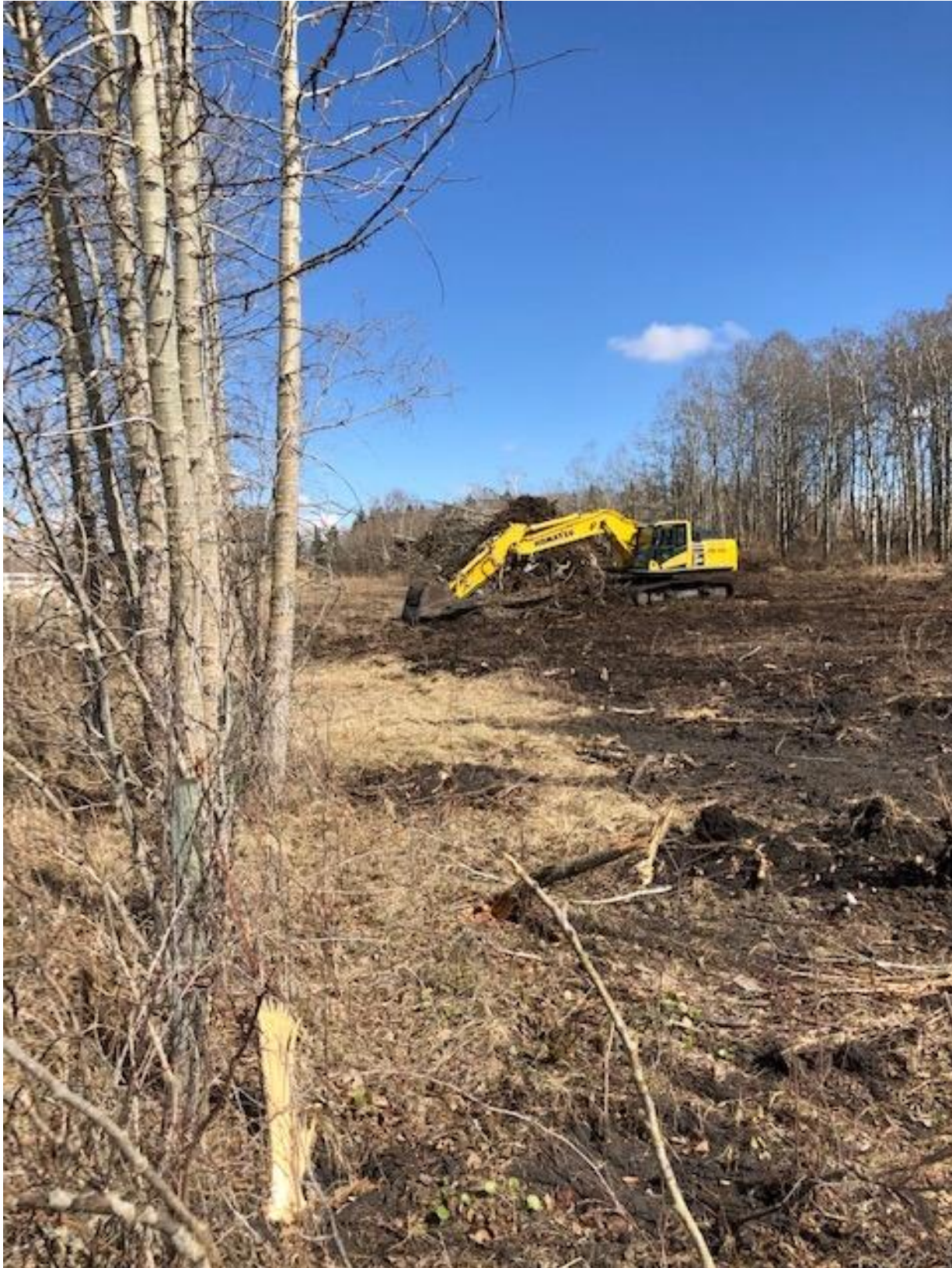
Stripping right to the property line
