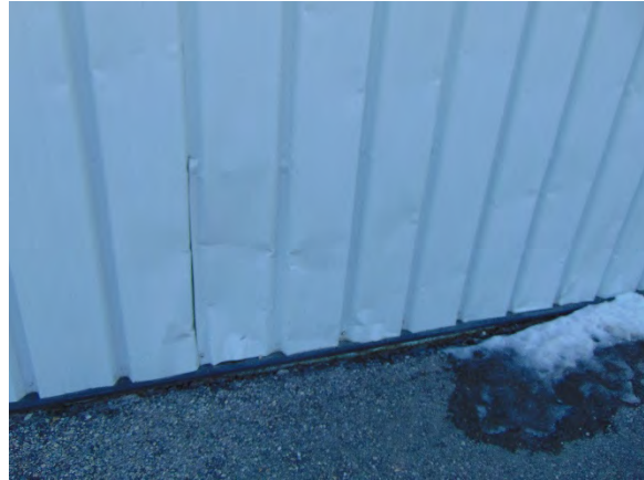
Photo 18 Impact damage at the exterior metal cladding
