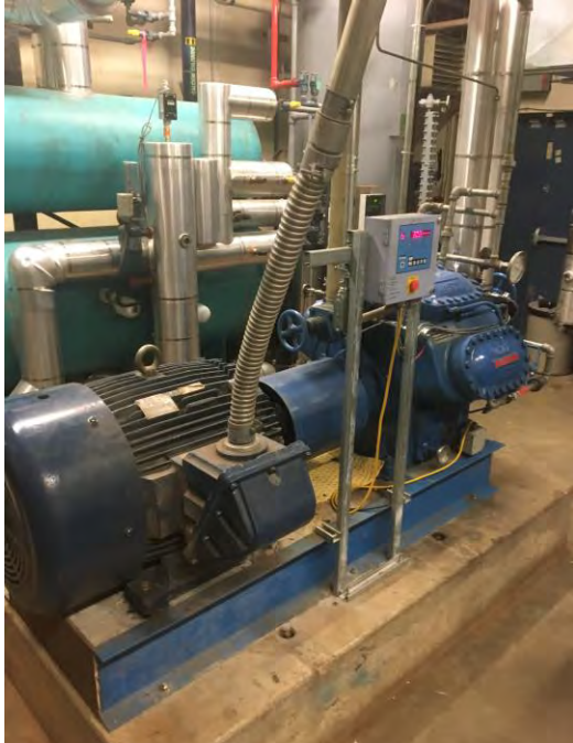
5. Compressor CM-201 showing Mypro temp wiring
