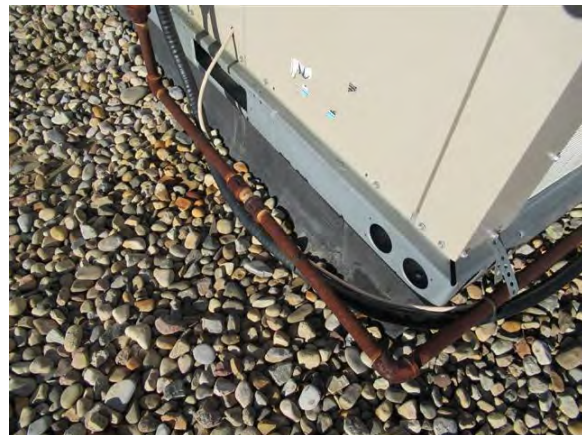
Photo 28 Deteriorated natural gas piping on the roof of the Curling Centre serving a roof top unit
