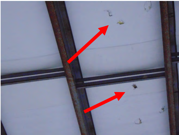
Photo 25 Impact damages at the Joe Phillips Arena's roof insulation
