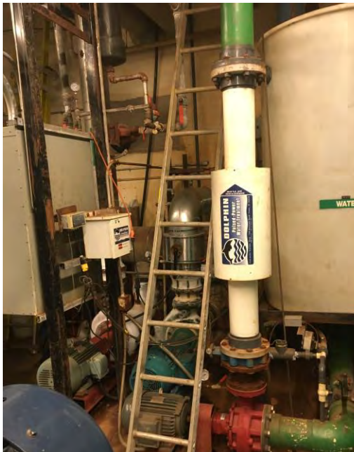
7. Dolphin water treatment, condenser pump and ladder access to expansion tanks
