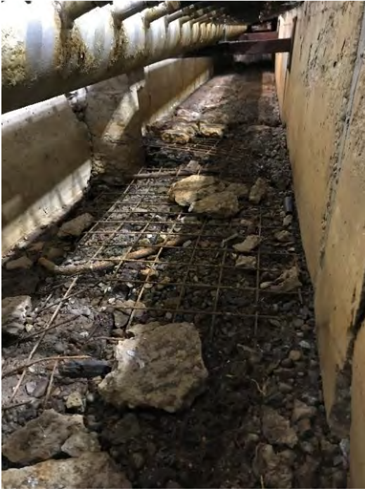
Photo 1. Red Dutton header trench floor condition
