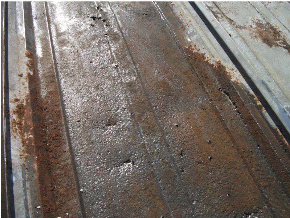
Photograph # 8: Corrosion through seams
