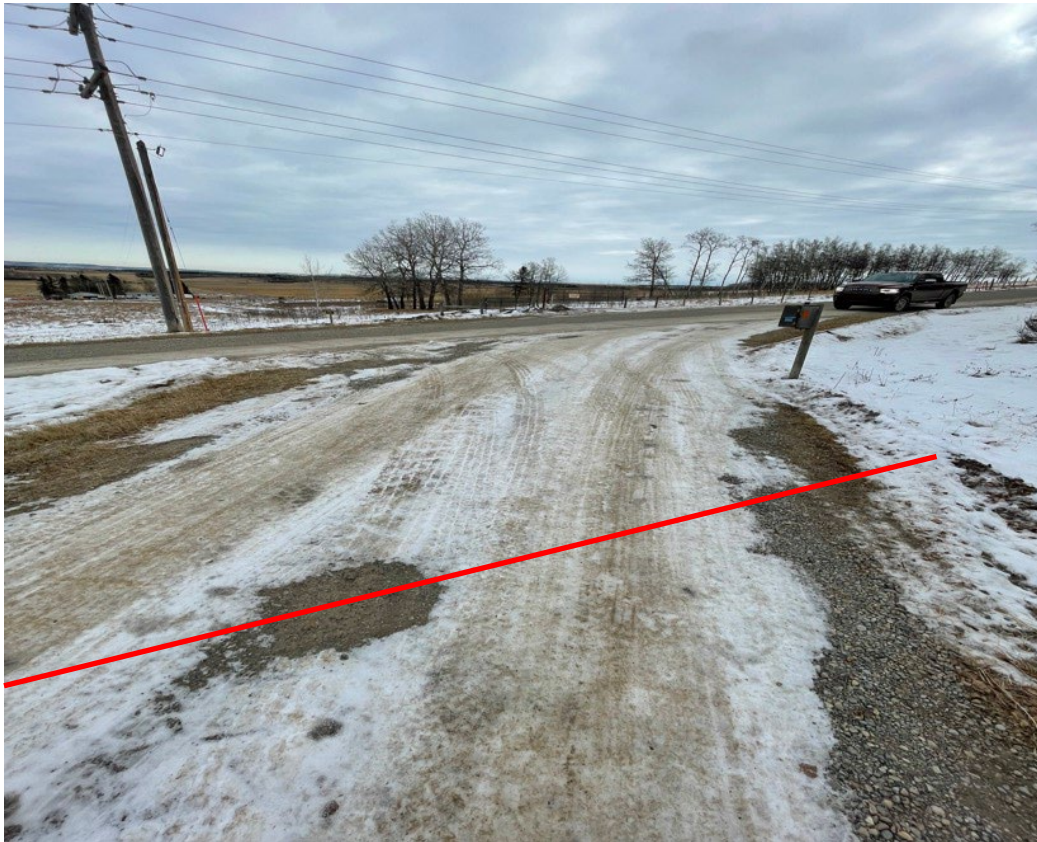
Leaving our property. Shallow ditch. Culvert installed by us.
