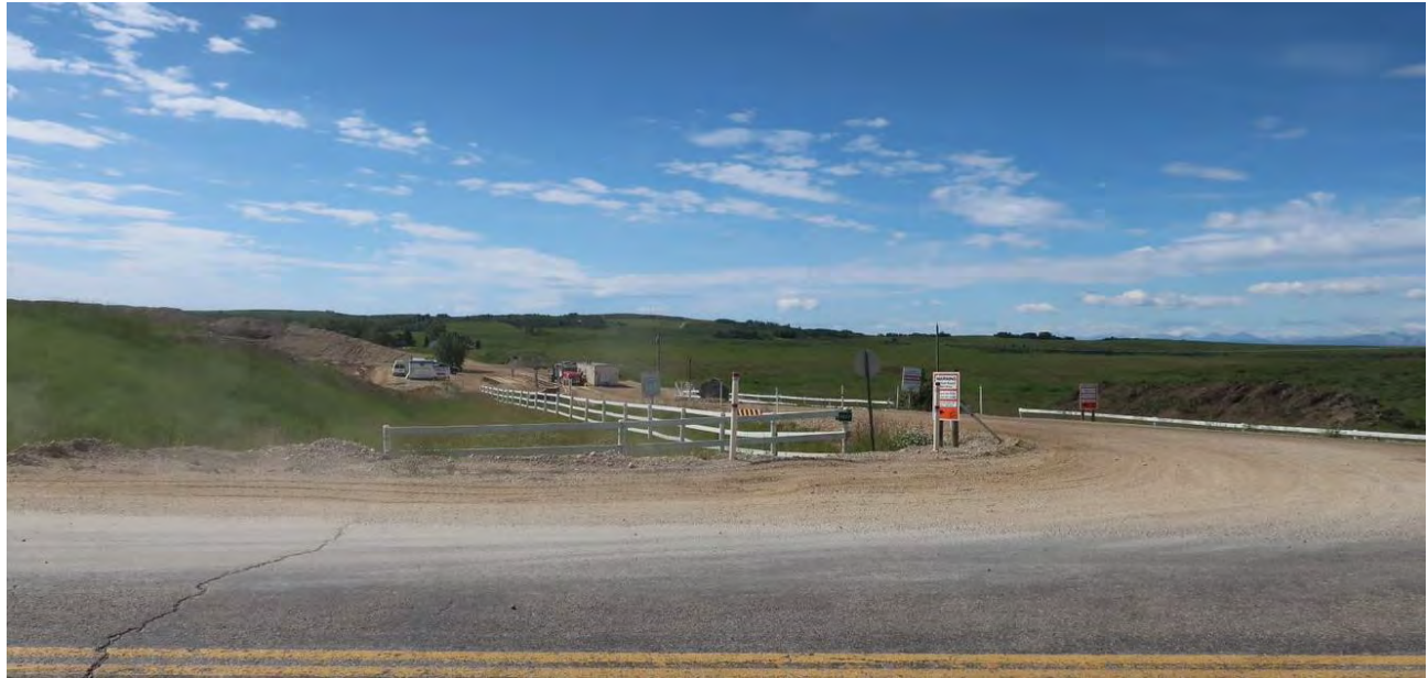
Figure 8 - View from the Hwy 567 to southwest (current access)
