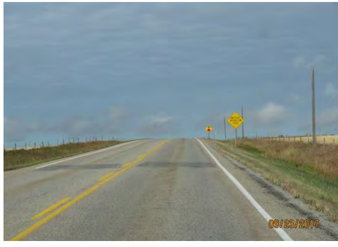
Photo 10: approaching intersection with poor intersection sight distance.
