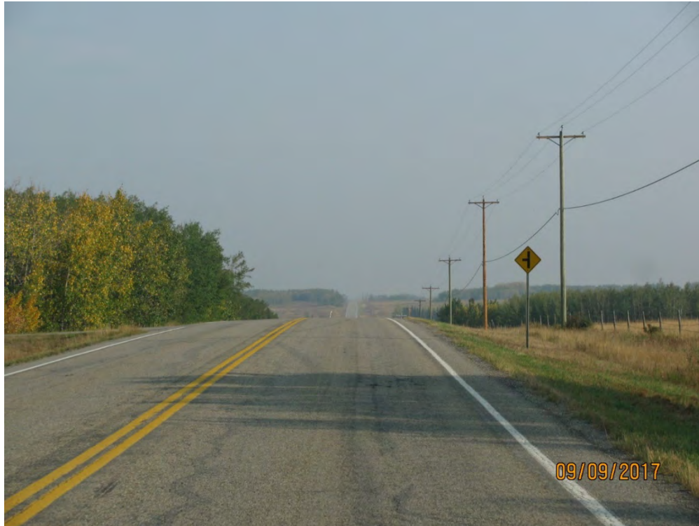
PHOTO 1 Hidden Intersection Hwy 776
