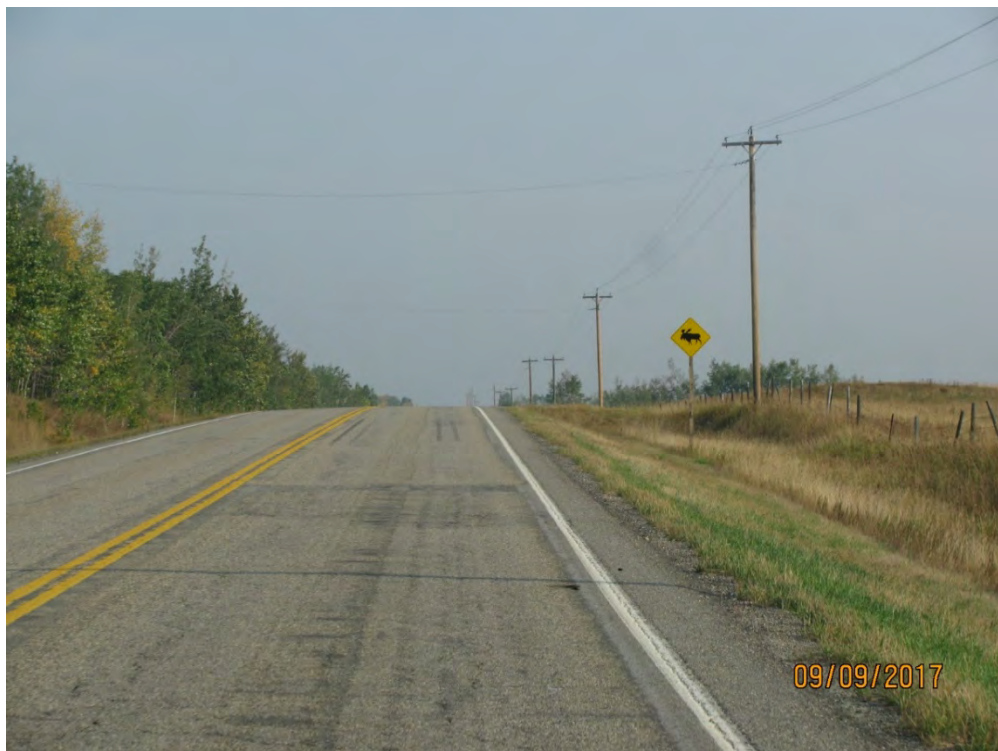
PHOTO 2 Wildlife Crossing Hwy 766
