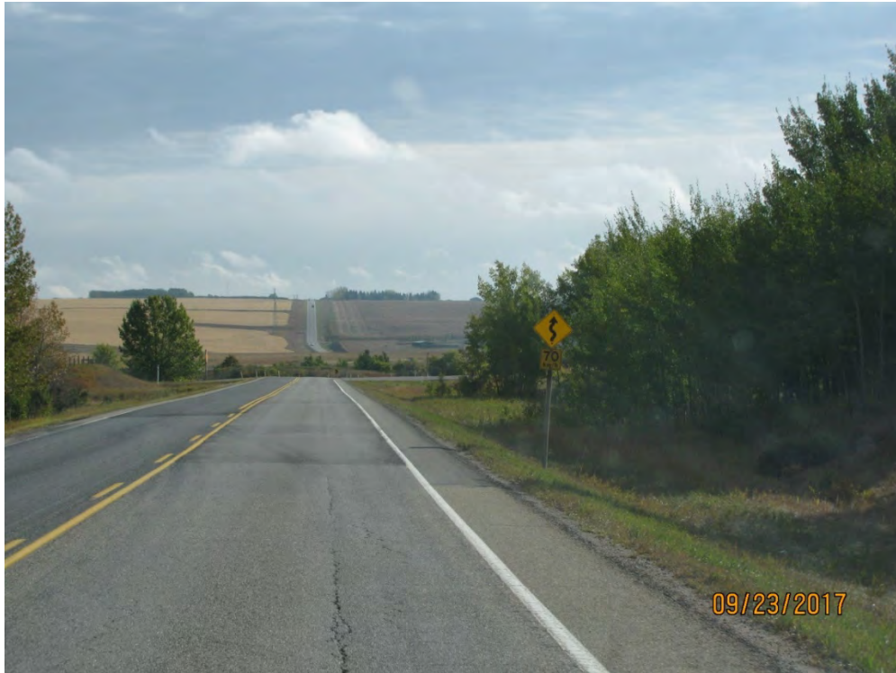
PHOTO 21 Hunt Coulee Hwy 567 EB
