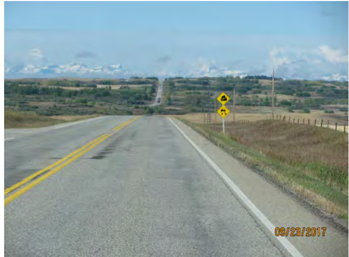
Photo 7: approaching large sag curve, Hwy 567.
