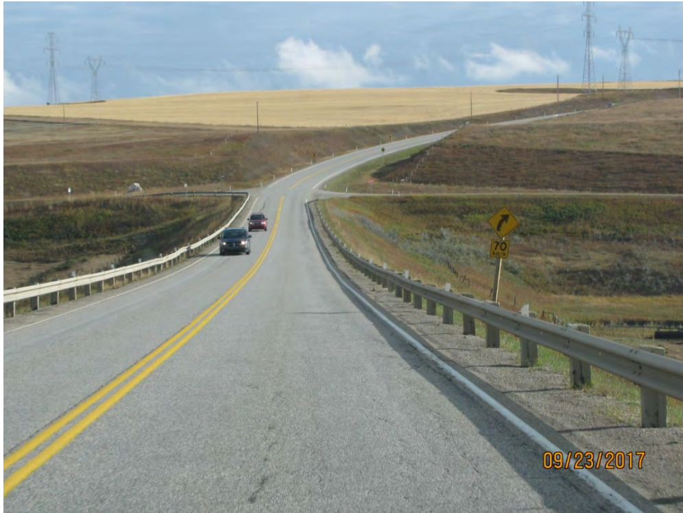
PHOTO 23 Hunt Coulee Hwy 567 EB
