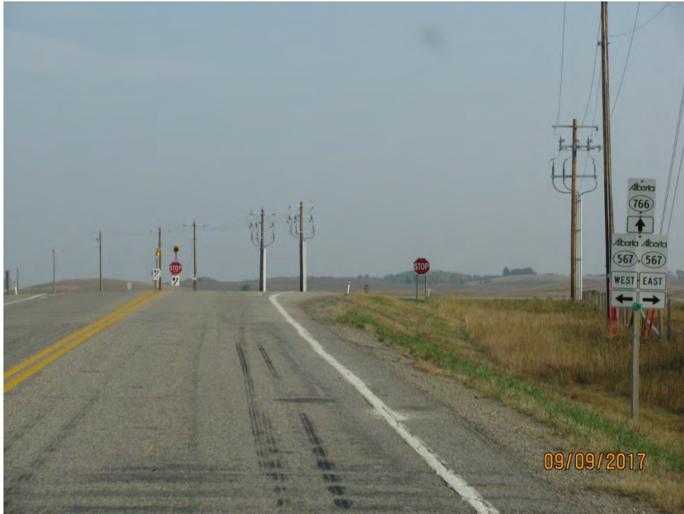
PHOTO 3 Junction Hwy 766 &amp; Hwy 567
