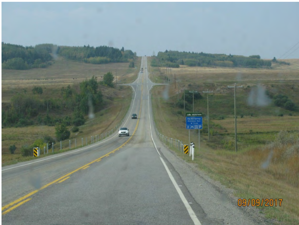
PHOTO 20 Hwy 567 Big Hill Springs Intersection
