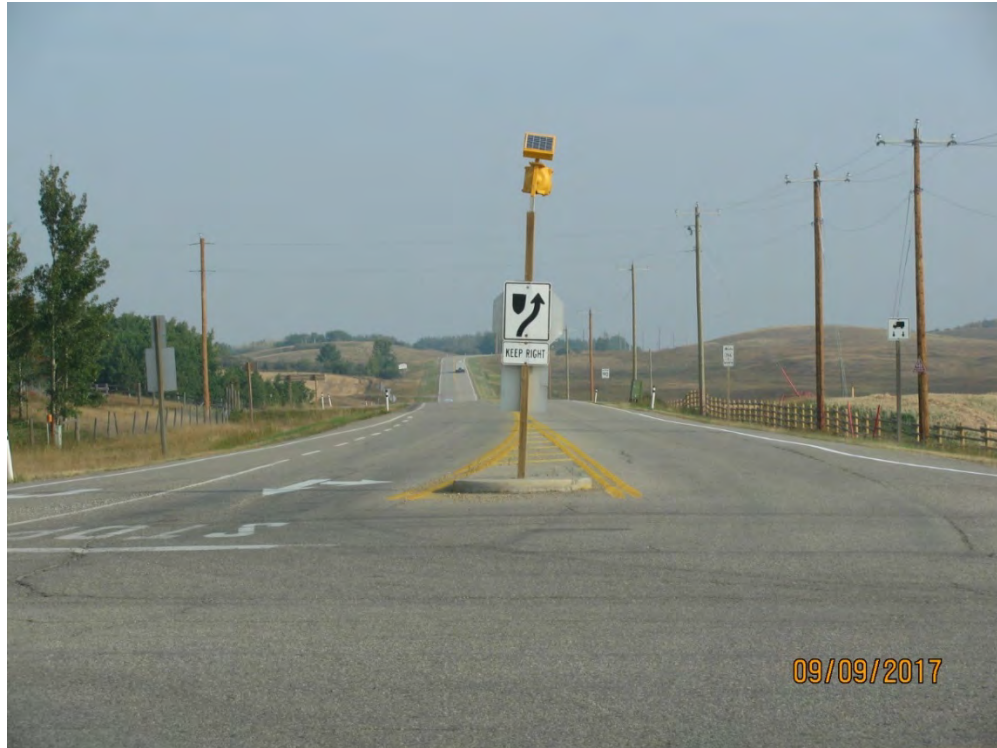
PHOTO 5 Junction Hwy 766 &amp; Hwy 567
