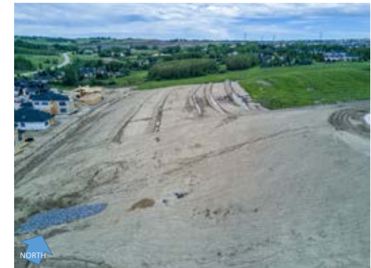
Existing Site Photos
