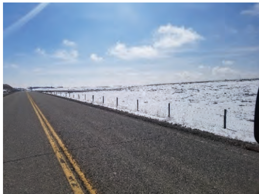
View facing South showing the fence marking the East property line.
