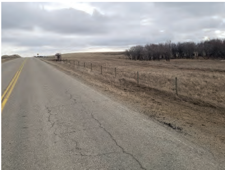
ENTRANCE TO OLSEN PIT FROM RGE RD 264 LOOKING SOUTH
