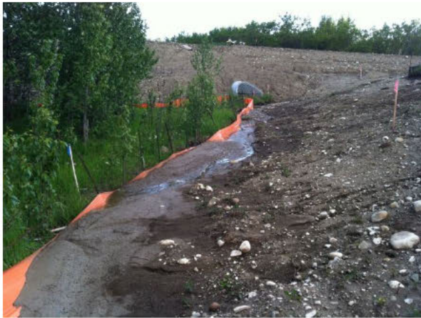
Figure 2. Photo taken on June 18 2013 , showing a drain installed by Silverhorn that channels storm water flow directly towards Equestrian Estate. This photo also highlights the level of erosion created by Silverhorn when they removed an extensive amount of trees and vegetation.
