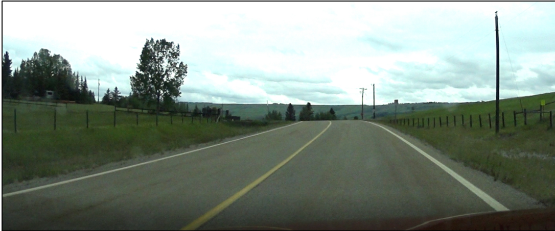
Figure A-5: Northbound Drive Through Vertical Curve Sight Distance
