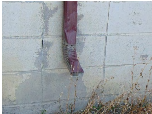
Photo 16 Missing rain water leader along the east side of the Main Facility
