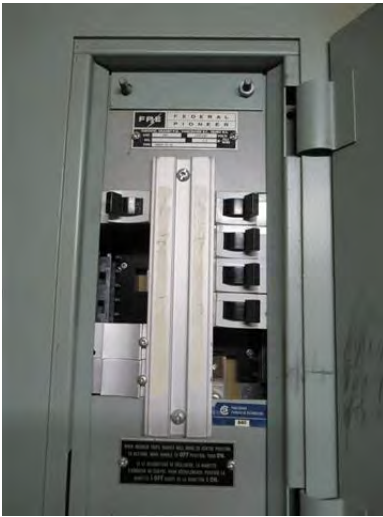
Photo 39 View of missing cover plates on panelboard in the Red Dutton Mechanical Room
