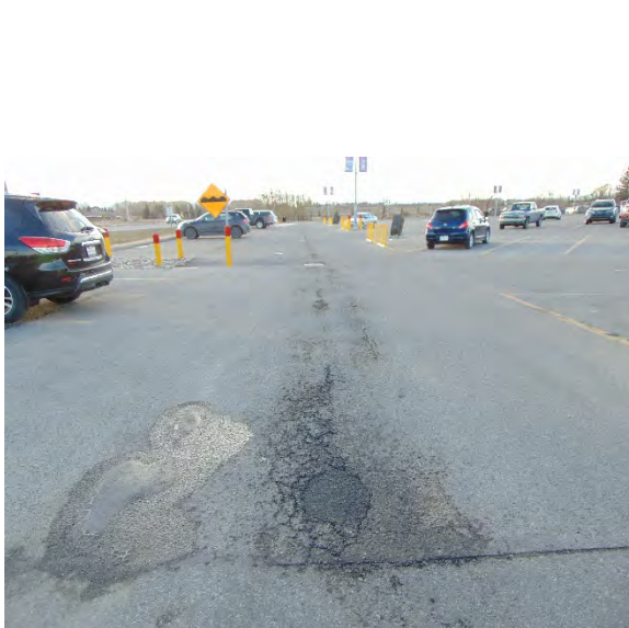
Photo 3 Typical condition of the asphalt paving at the south parking lot
