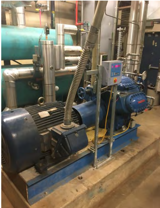
5. Compressor CM-201 showing Mypro temp wiring
