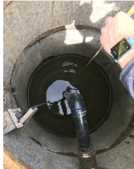
Photo 5. Water level in French drain collector sump manhole with failed pump
