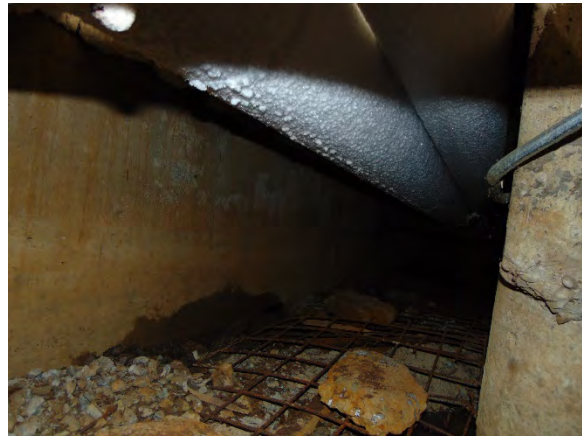
Photo 12 Exposed rebar and debris in the Red Dutton Arena header trench
