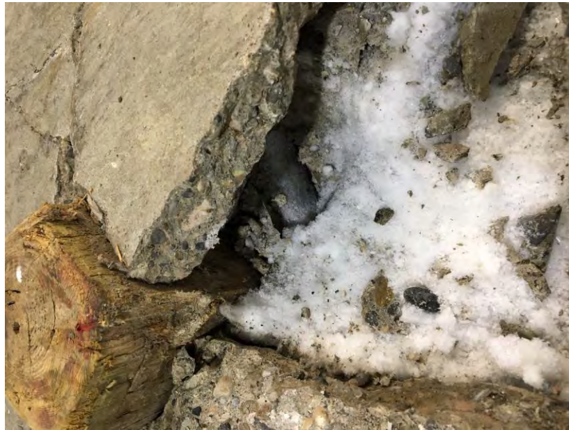
Photo 3. Slab condition and ice formation under slab adjacent to Red Dutton Arena
