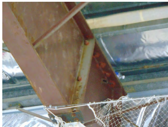
Photo 10 Surface rust and rusty bolt connections on the Red Dutton Arena
