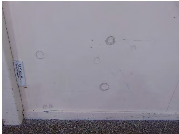
Photo 24 Impact damages in the Shane Homes Curling Rink's plywood siding.
