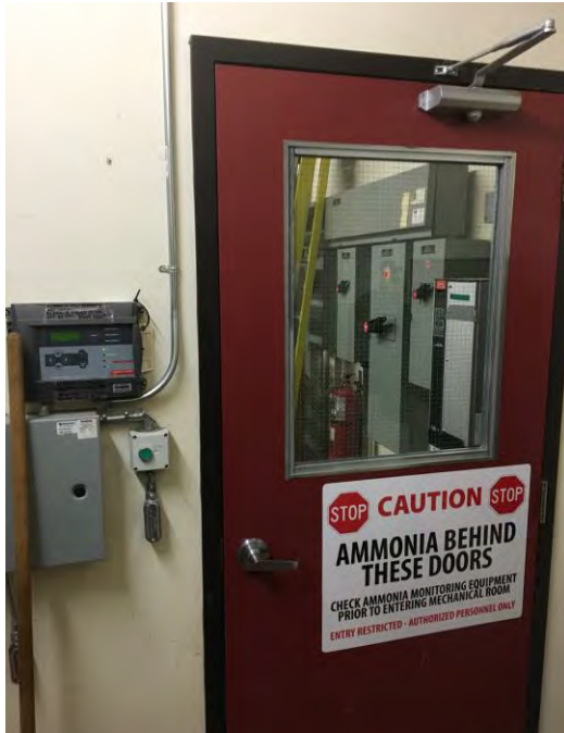
1. Vestibule door with NH 3 detection panel and ventilation fan on switch
