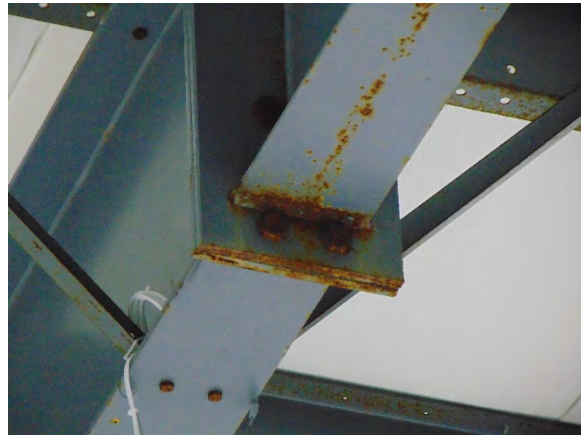
Photo 8 Surface rust and rusty bolt connections and head plates in the Joe Phillips Arena
