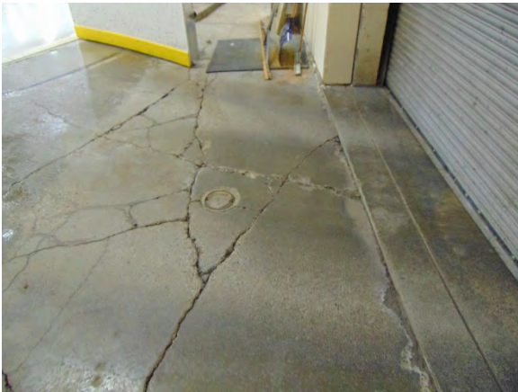
Photo 13 Failed concrete slab section at the Zamboni "driveway" in the Red Dutton Arena
