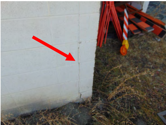
Photo 19 Cracking observed along the east side of the Main Facility
