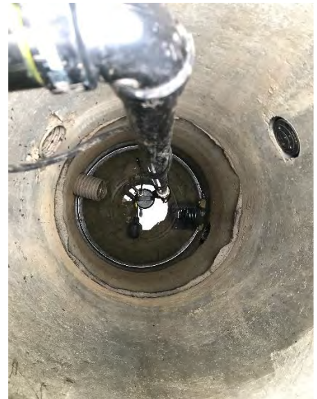
Photo 7. French drain collector sump with pump operational
