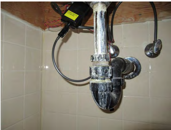
Photo 27 View of previous water leak under lavatory in one of the change rooms
