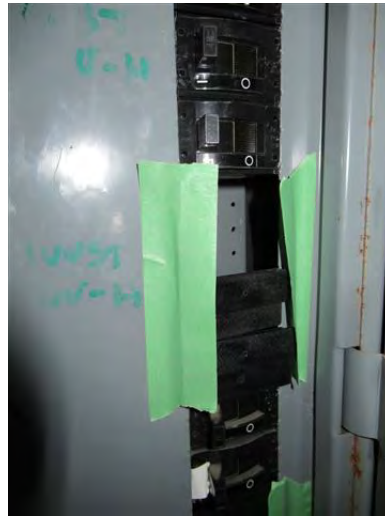
Photo 40 View of another missing cover plate on circuit breaker in Refrigeration Room
