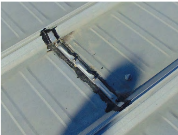
Photo 15 Repaired roof section on the Joe Phillips Arena
