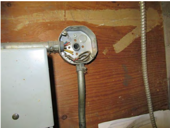
Photo 43 Missing cover plate on junction box in Red Dutton Mechanical Room
