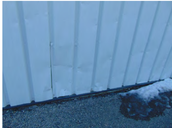
Photo 18 Impact damage at the exterior metal cladding
