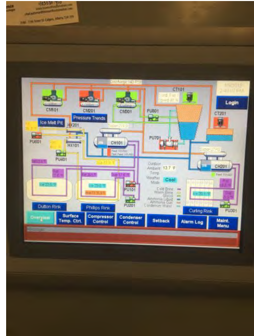
2. PLC system flow screen
