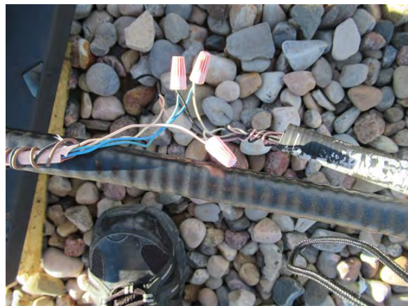
Photo 42 Exposed controls wiring on the roof of the Curling Centre
