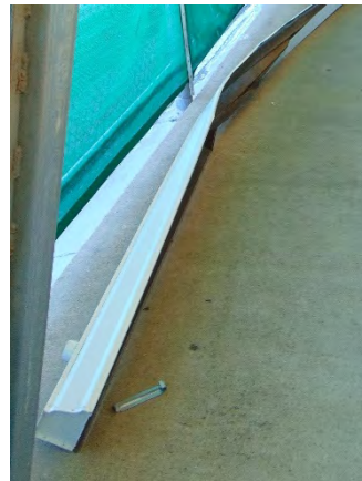
Photo 20 Damaged rainwater gutter at the Outdoor Rink
