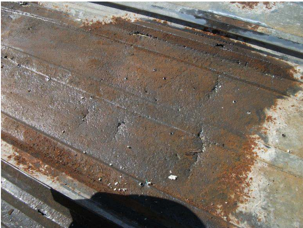
Photograph # 6: Metal is weak, numerous perforations
