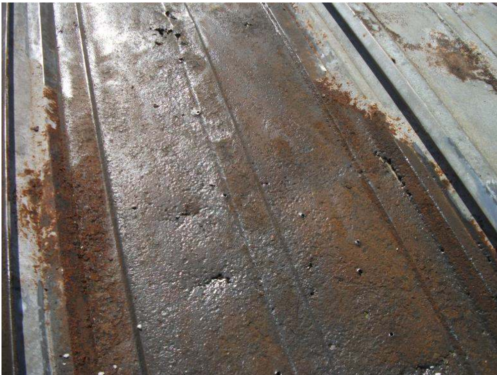
Photograph # 8: Corrosion through seams
