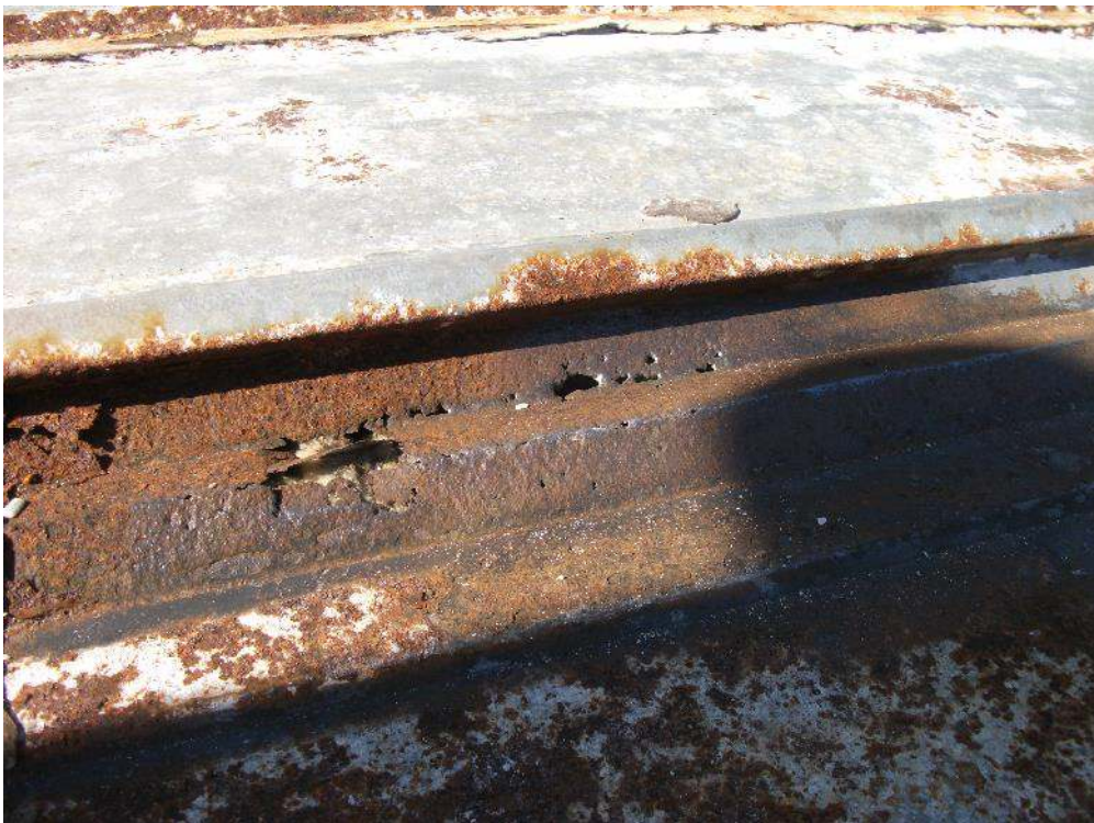
Photograph # 4: Holes in panel
