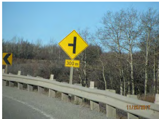
Photo 5: hidden intersection following horizontal curve on Hwy 567.
