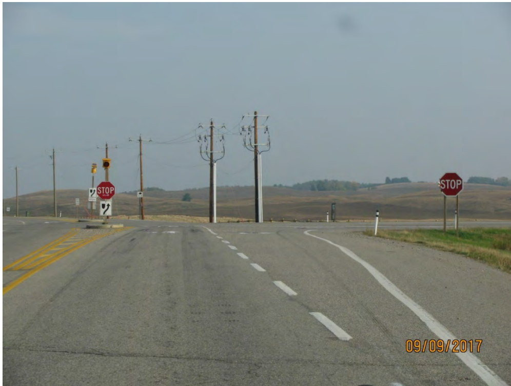
PHOTO 4 Junction Hwy 766 & Hwy 567
