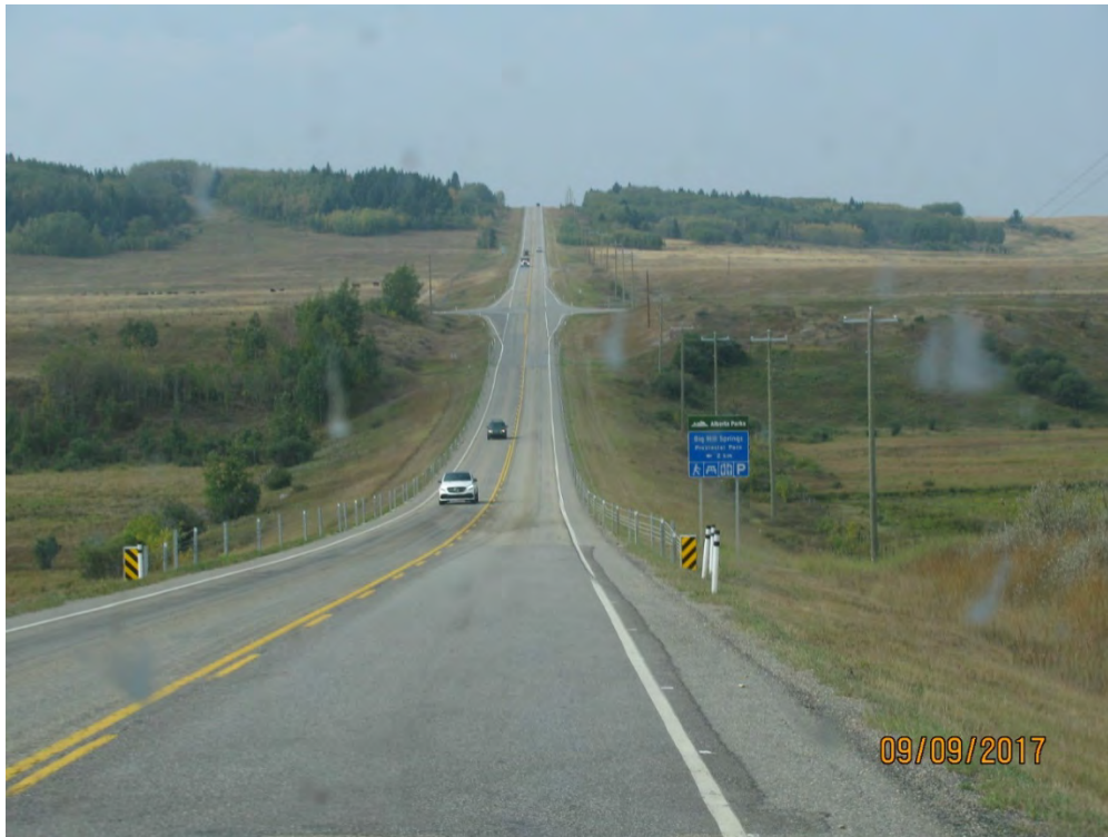
PHOTO 20 Hwy 567 Big Hill Springs Intersection
