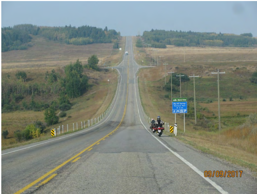
PHOTO 8 Scooters on Narrow Shoulder of Hwy 567
