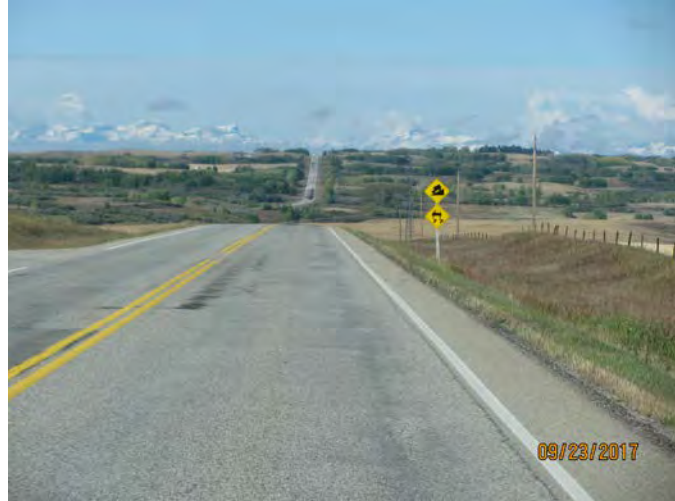
Photo 7: approaching large sag curve, Hwy 567.
