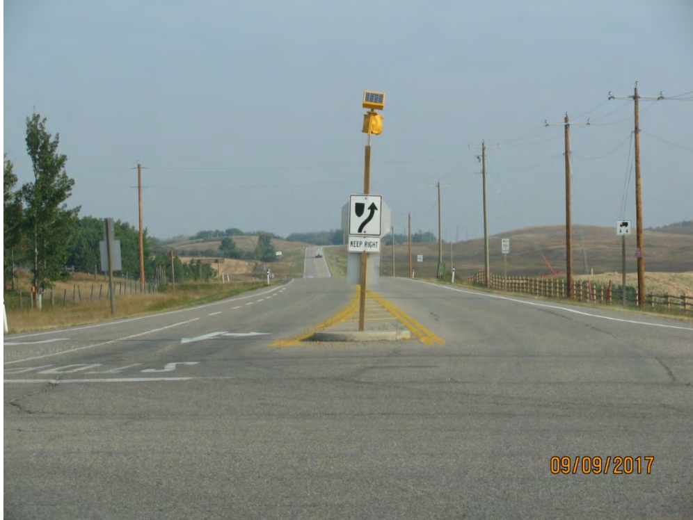
PHOTO 5 Junction Hwy 766 & Hwy 567
