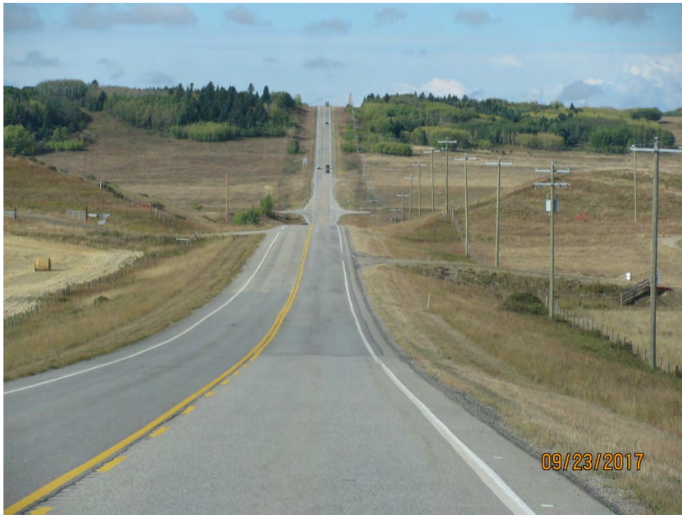
PHOTO 32 Hwy 567 WB – Long Sag Curve
